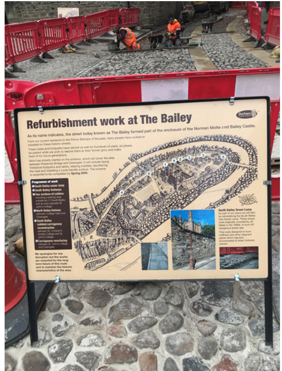
Refurbishment of the Baileys using traditional river cobbles
